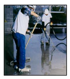
Pour Today, Place Floor Goods Tomorrow. Level-Right, Lever-Right PLUS and Level-Right FS-10 help keep your job on the fast track with installation of finished floor goods just hours after the pour. Ceramic tile can be thin set within 2 to 4 hours. Other floor goods can be installed once Level-Right, Lever-Right PLUS or Level-Right FS-10 pass a moisture test.
